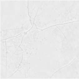
Cracked white 20MM
